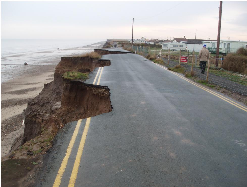
Figure 6.1 Coastal Erosion affecting Roads in the East Riding
