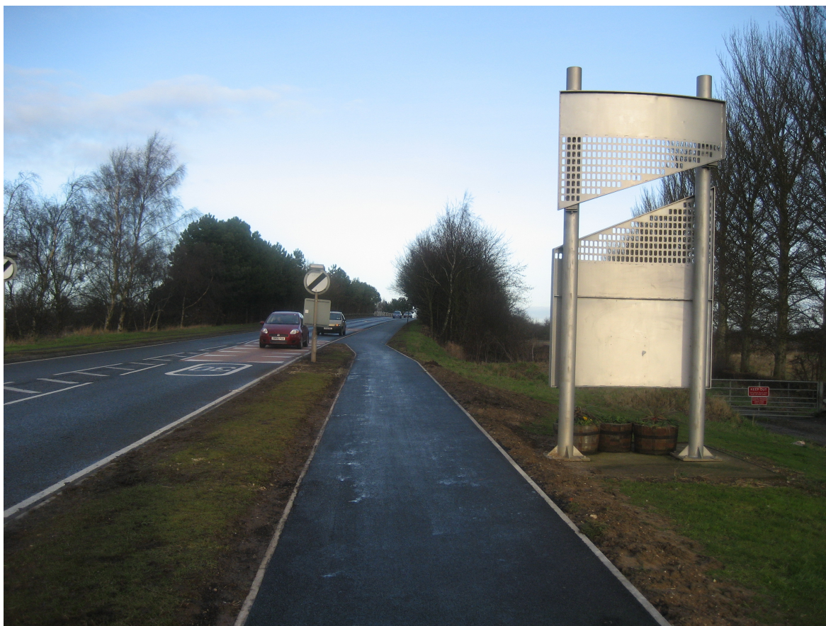
Picture 15.1 The New Off-Road Cycle Route Between Goole and Howden
