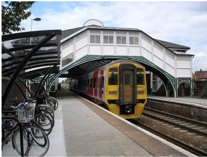
Figure 18.4 Covered Cycle Parking and Footbridge Renovation at Beverley Station
