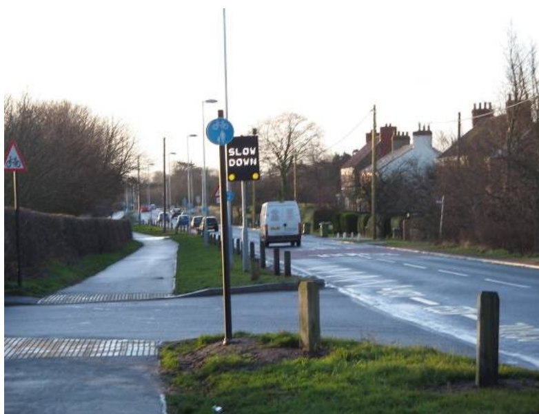
Figure 22.1 Vehicle Activated Signs on Station Road between Hedon and Preston
